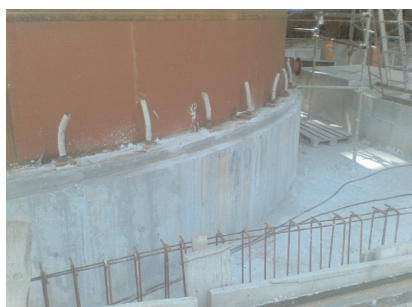
TE Šoštanj: after grouting with Tekamal Alteks SCC 0-3
