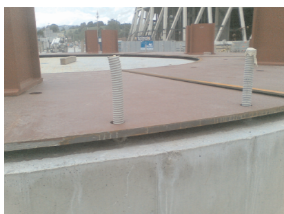
TE Šoštanj: before grouting with Tekamal Alteks SCC 0-3
