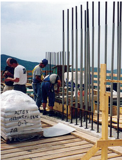
Viaduct Črni Kal - pouring of structural bearings
