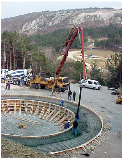
Fountain at the column on viaduct Črni kal.
